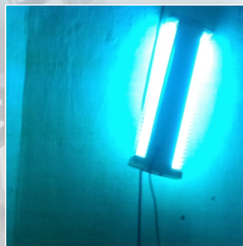
A Specialty Developed ultra Violet radiator is used to remove all types of micro organism present in the tank
