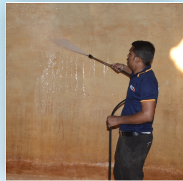
Specially developed antibacterial agent is spread by high pressure jet throughout water tank to remove various bacteria
